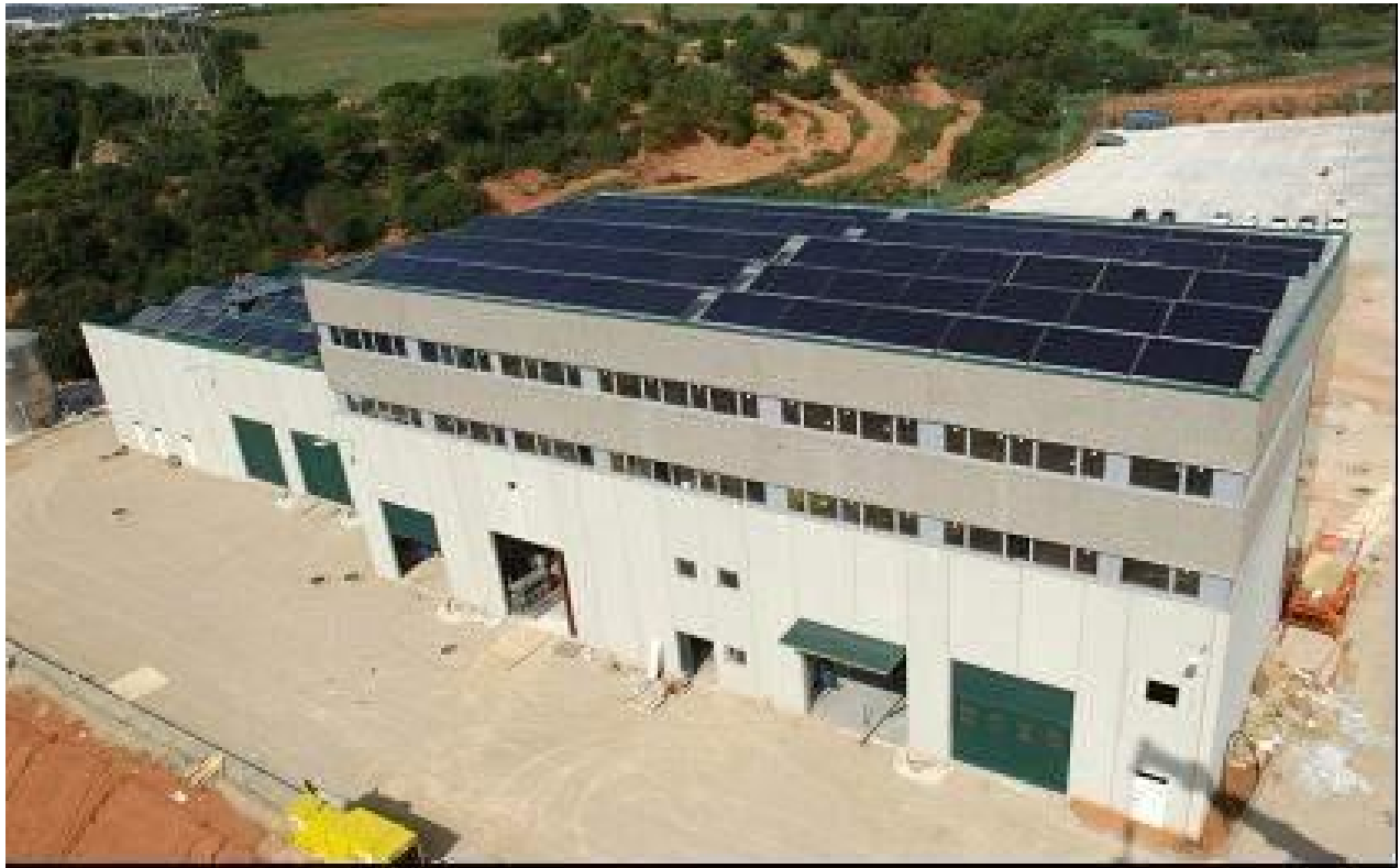
Parking service Castellbisbal SA, container washing, Barcelona, Spain. Installed capacity: 357 kWth. Source: Aiguasol Engineering, Spain.
